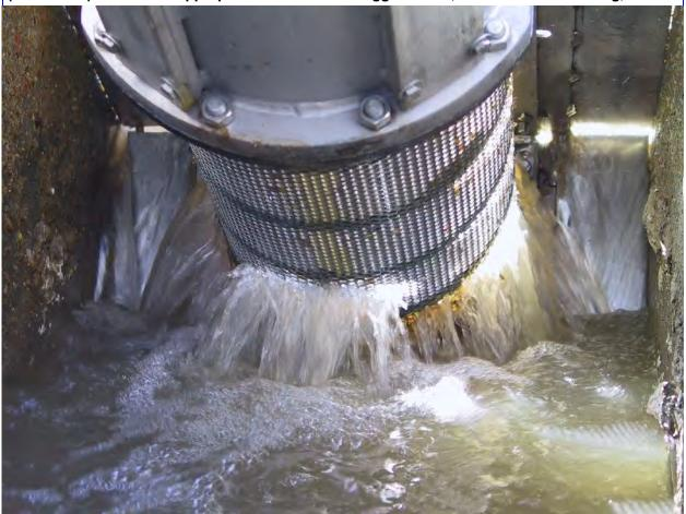
starts washing, and this is the result. In this shot, there is some spill over the barriers on the sides. They've adjusted the trigger level so that doesn't happen any more. From experience, there's a definite improvement in the visual quality of the influent. No more chunks of grease and rags downstream. The grit is cleaner too, with far less organic material in it. In fact, we think a lot of the grit is being twisted up into the rags and mop strings.
