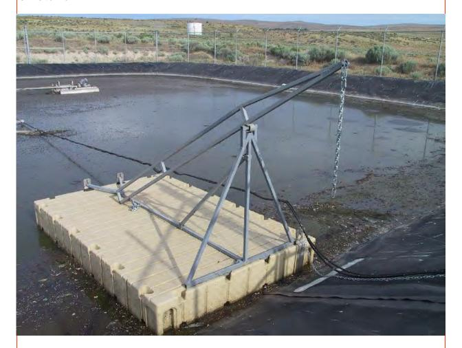
Recognize the origin of the lifting device? Yes, it's salvaged from a utility truck rack normally used to transport pipes, ladders, lumber, etc. There's another view of it on the next page.
