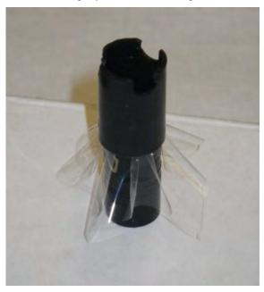
Trim excess membrane with scissors or a sharp blade.
