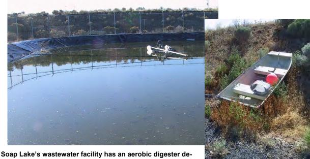
signed like a mini-lagoon with surface aerators. Here's a shot one corner of it (above left). The power and anchor cables go across in this photo. One of two surface aerators is shown at idle for decanting.
