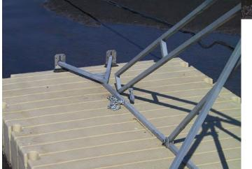
Notice the hook and chain at left for suspending the load.
