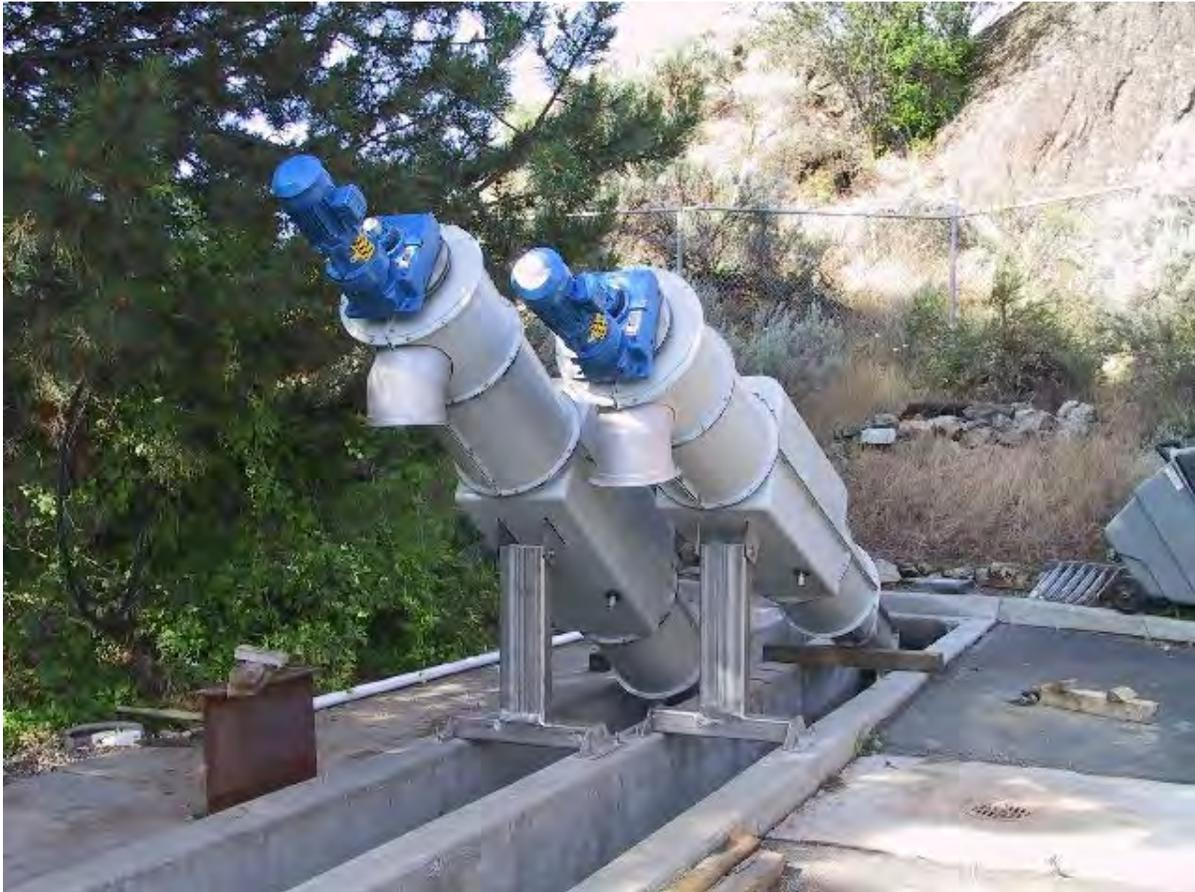
The unit on the right is propped up over the active influent channel. The left side one is sitting on the bottom of the inactive channel, preparatory to adding channel seals. Grit removal is not included in this project, so the operators will still have to hand-shovel grit out of the grit traps downstream. But the grit should come out cleaner than in the past.
